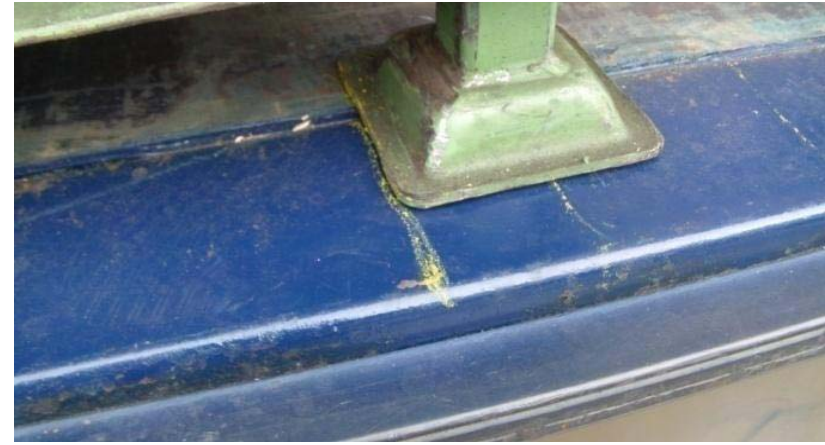
Position of the mesh pallet after the test, no shifting detectable
