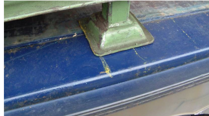
No further sliding after the test was detectable
