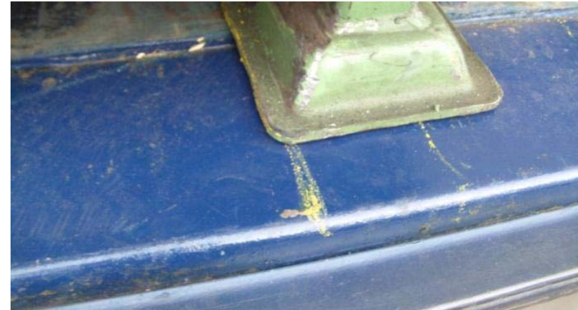
Position of the mesh pallet after the test, minimal shifting detectable
